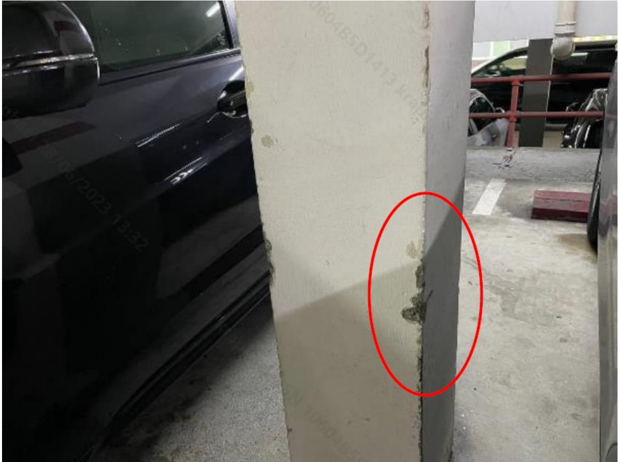
Figure B-6: Damage to Carpark Pillar
