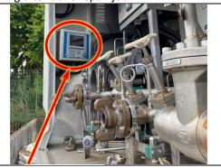
P5. Flow meter need to dismantle out / disconnect cable & install back / rewiring after done repair job
