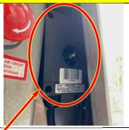
P7. EX proof on-off switch for light need to dismantle out / disconnect cable & replace with new / rewiring after done repair job
