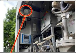
P6. EX proof light need to dismantle out / disconnect cable & install back / rewiring after done repair job
