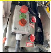
P8. Motor remote on /off switch & valve control air switch need to dismantle out / disconnect cable & install back ( May be need to repair ) / rewiring after done repair job
