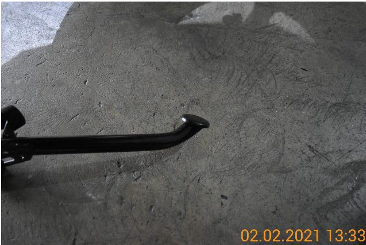
162/181: Post Repair Photo
