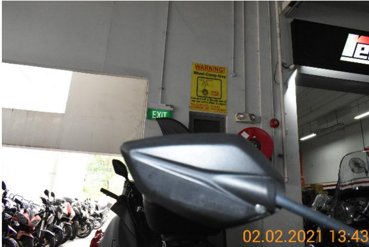
167/181: Post Repair Photo
