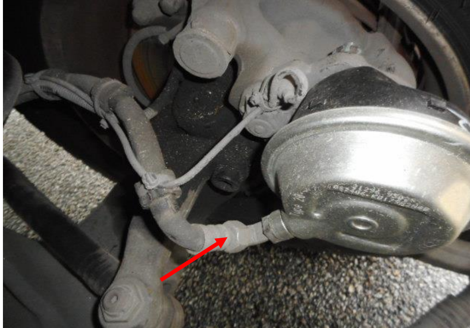
Photo 18 shows the brake pipe (arrowed) at the front right wheel of the Motor Bus. I did not observe any leakage of brake fluid at the time of my inspection of the Motor Bus. My static tests of the Motor Bus's braking system, along with my visual examination of the various mechanical components in the braking system, had indicated that there was no internal leakage of pressure/vacuum. Hence the braking system of the Motor Bus was likely to be in serviceable condition at the material time of accident.
