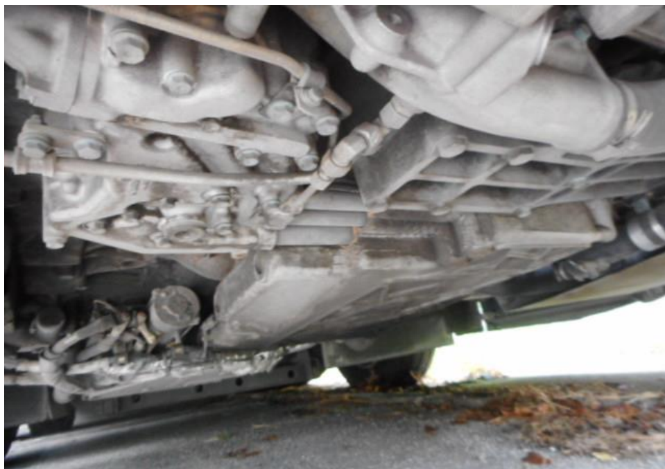
Photo 23 shows the undercarriage of the Motor Bus, at the area where the engine housing and transmission housing are located. I did not find any sign(s) or indication(s) of fluid leak and/or fluid stain(s) on the underside of the Motor Bus.
