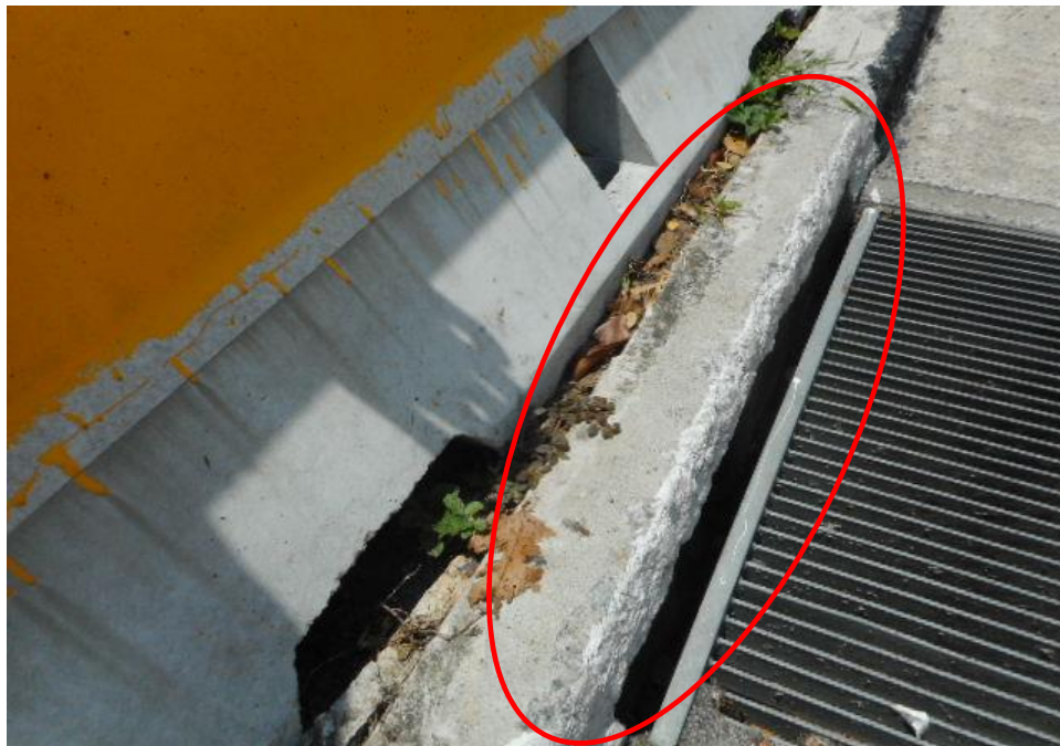
Photo 10 shows the close up view of the curb side, the curb had suffer damaged as a result of the Insured Vehicle mounting it (circled). In general, the information that could be gathered from this photograph had corresponded to the events that were related to us by Mr Lau, location when the accident happened.
