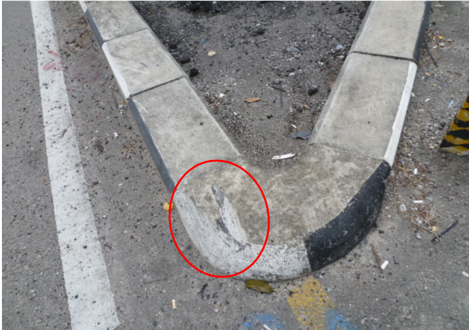
Photo 3 shows the graze marks and tyre marks found on the kerb which Ms Pek had mounted (circled).
