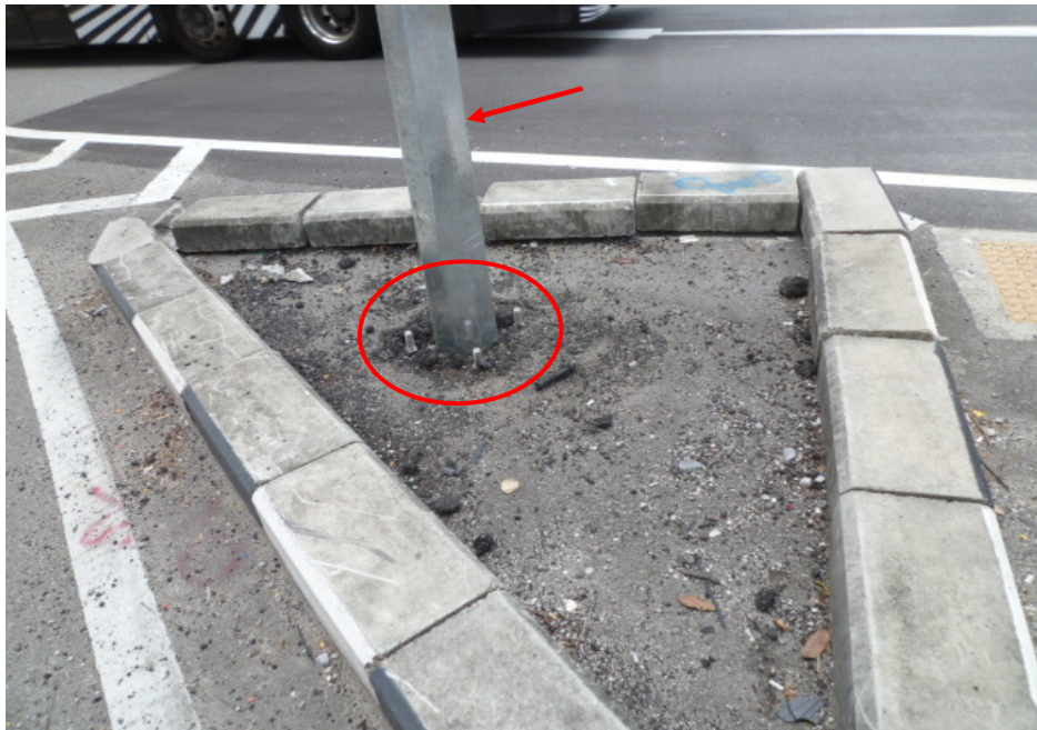
Photo 5 shows the lamp post (arrowed) which Ms Pek had collided into. We observed that the base of the lamp post had been replaced. The bolts surrounding the base of the lamp post and the re-laid tar are indications that it had been recently replaced (circled).
