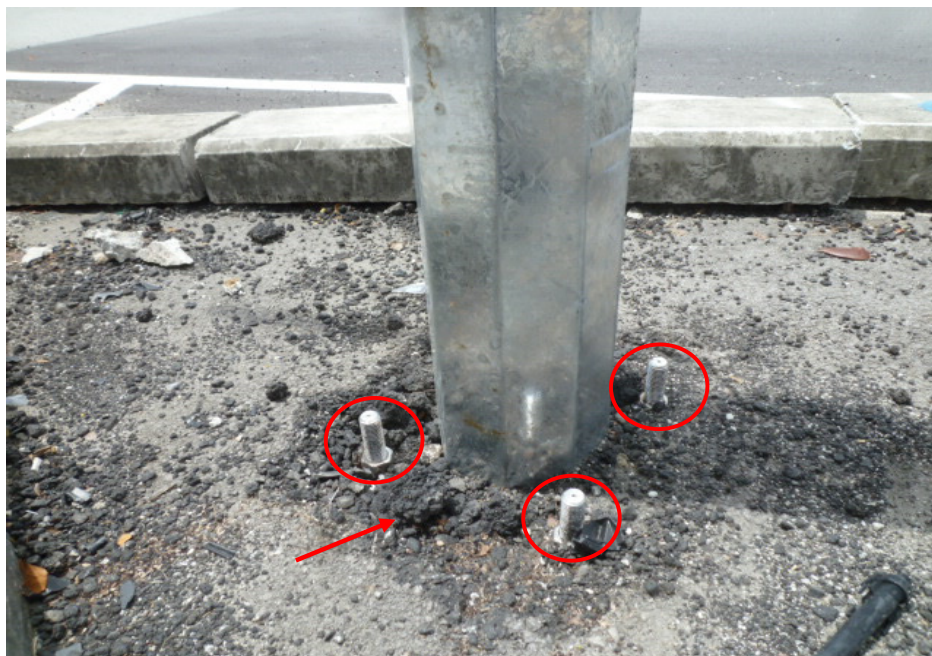
Photo 6 shows a close up view of the bolts surrounding the base (circled) and the re-laid tar (arrowed) at the bottom of the lamp post which are indications that the base of the lamp post had been recently replaced.
