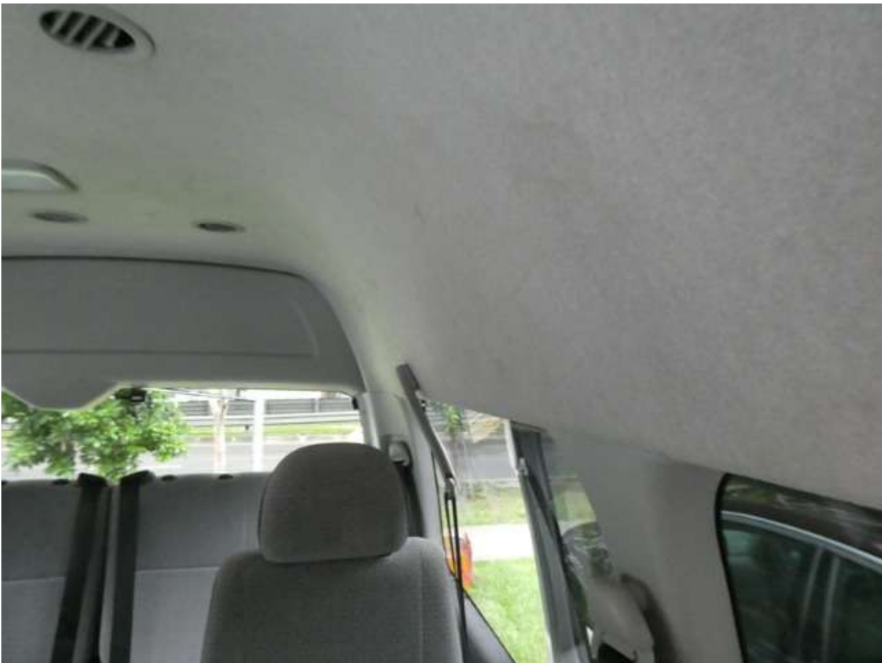
275/284: After Repair Photo
