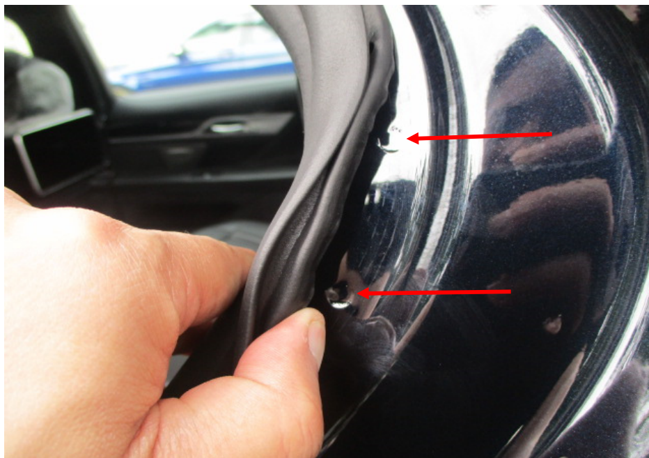
Photo 28 shows the left side "C" pillar of the Motor Car. I did not find any weld marks other than original spot weld marks (arrowed) on the left side "C" pillar of the Motor Car which, indicates that there was no re-welding works carried out. In general, I had found all the non-detachable body panels of the Motor Car to be originally fitted at the time of my inspection.
