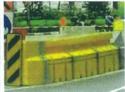
Use of crash cushion to shield the leading terminal of the concrete safety barrier
