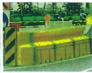
Use of crash cushion to shield the leading terminal of the concrete safety barrier
