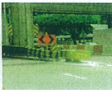
Use of crash cushion to shield the leading terminal of the w-beam VIG
