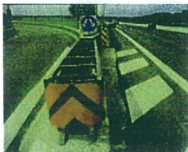
Example of a stationary attenuator system
