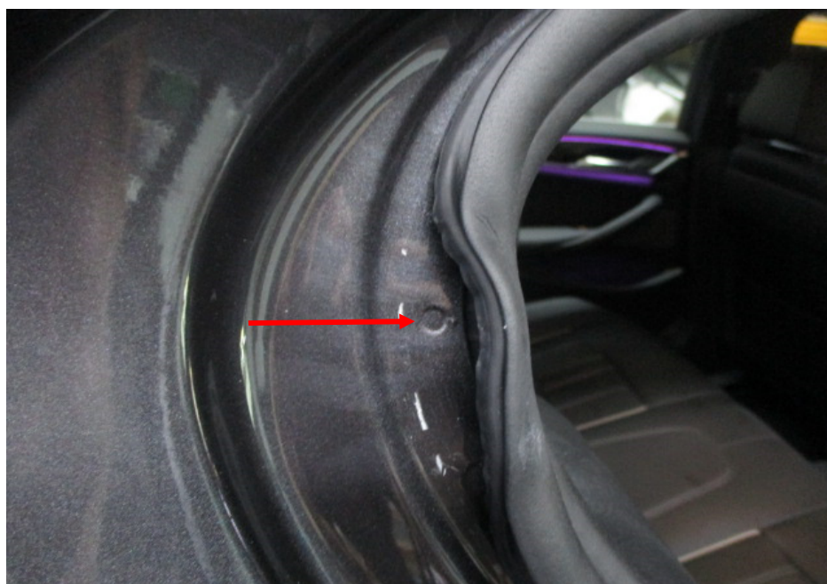
Photo 31 shows the right side "C" pillar of the Motor Car. I did not find any weld marks other than original spot weld marks (arrowed) on the right side "C" pillar of the Motor Car which, indicates that there was no re-welding works carried out. In general, I had found all the non-detachable body panels of the Motor Car to be originally fitted at the time of my inspection.
