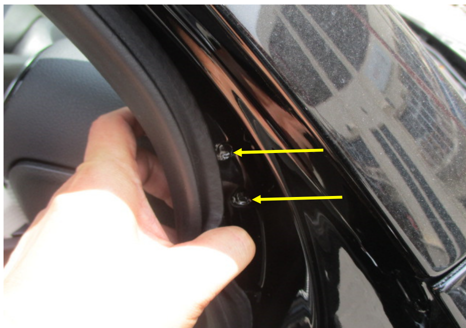
Photo 25 shows the right side "A" pillar of the Motor Car. I did not find any weld marks other than original spot weld marks (arrowed) on the right side "A" pillar of the Motor Car which, indicates that there was no re-welding works carried out. In general, I had found all the non-detachable body panels of the Motor Car to be originally fitted at the time of my inspection.
