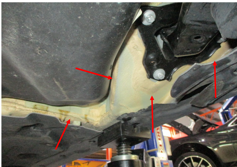
Photo 19 shows the floorboard and chassis/structural body at the underside rear right of the Motor Car. The original factory sealant (arrowed) at the joints between the floorboard and along the chassis/structural body was observed to be untouched. In general, I had found no work was carried out on floorboard and on the chassis/structural body of the Motor Car.
