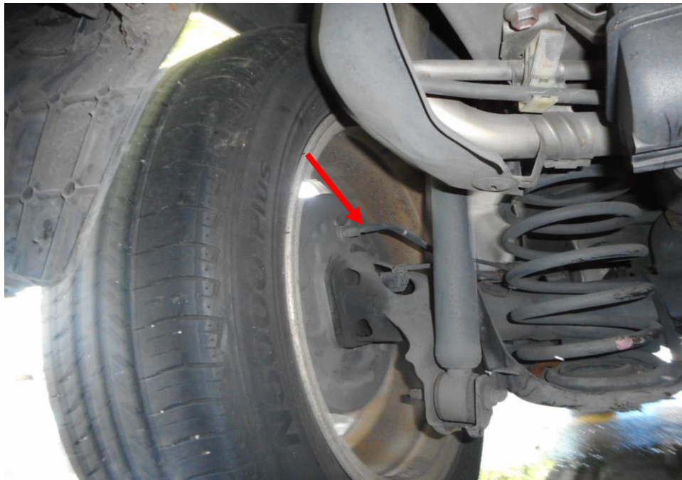
Photo 18 shows the brake hose/pipe (arrowed) at the rear left wheel of the Motor Car. No leakage of brake fluid was observed. Visual examination of the various components of the braking system like the drum brake, brake booster, brake pedal etc. had revealed all to be intact and without visible damage.
