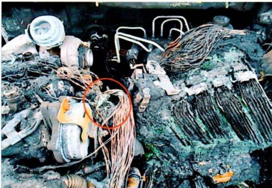
Photo 10 shows a closer view of the greenish residue found on some of the burnt stretches of original factory fitted wirings (arrowed). The presence of such greenish residue suggests occurrence of an electrical short circuit.
