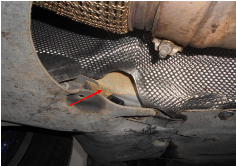
Photo 13 shows the floor board at the underside right front of the Motor Car. The original factory sealant (arrowed) at the joints along the non-detachable body panels were untouched, indicating no work was done on the non-detachable body panels of the Motor Car; and that these body panels were originally fitted.
