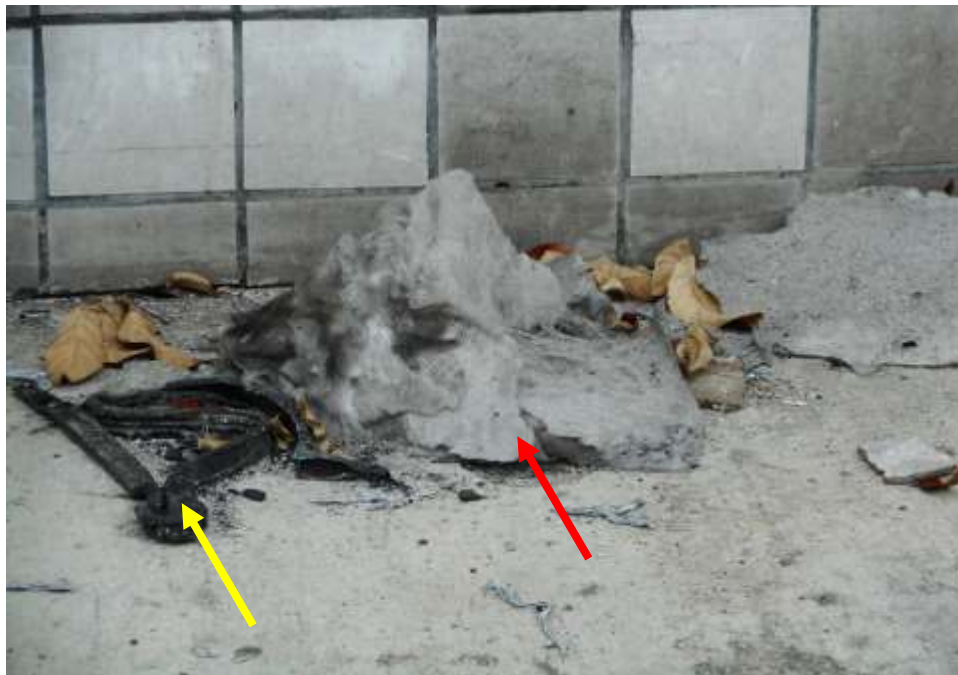
Photo 22 shows the traces of residue materials of the roof linings and melted parts from the Insured Vehicle. The roof linings materials (red arrow) and parts of the Insured Vehicle (yellow arrow) had fallen off the roof onto the ground due to the intensity of the fire.
