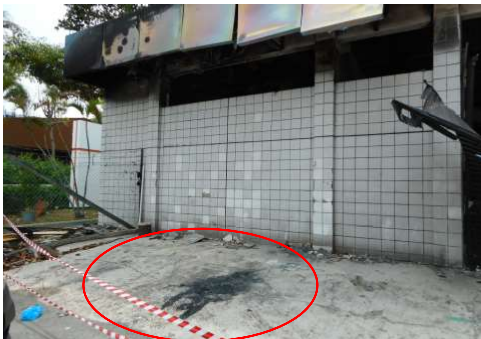
Photo 23 shows the general view of the location where the fire incident had occurred. The Insured Vehicle was positioned head in at the front pouch of the Rubbish Collection Centre at Chai Chee Lane Block 512. From our observations, we see a melted leftover black residue of plastic on the ground which was the melted air filter box from the cabin top of the Insured Vehicle. (circled) Due to the burning roof lining landed on the air filter box and melting it onto the ground.
