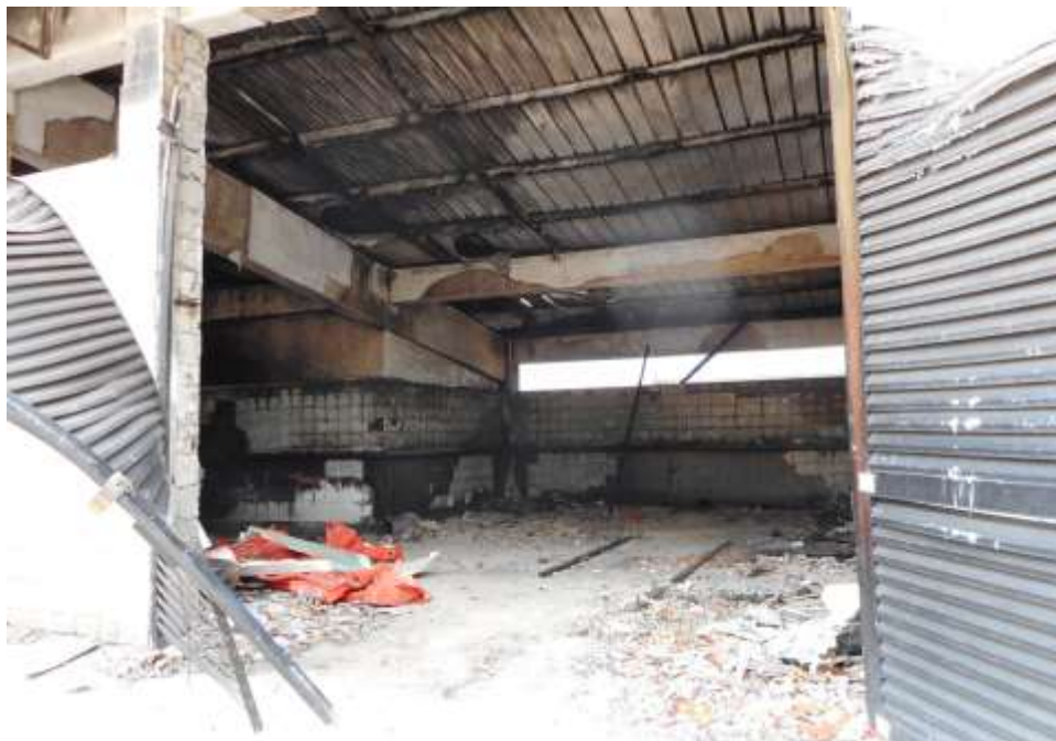
Photo 19 shows the close up view of the inside of the Rubbish Collection Centre at Chai Chee Lane Block 512. From our observations, the doors, walls, roof and surroundings combustible materials were affected by the fire.
