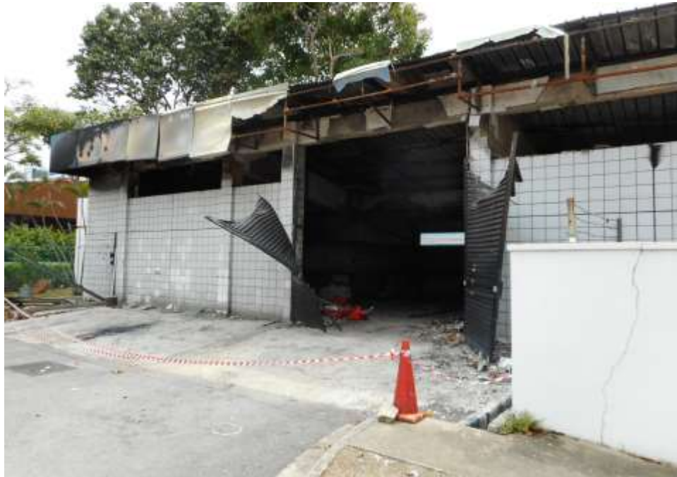
Photo 18 shows the general view of the location where the fire incident had occurred. The Insured Vehicle was positioned head in at the front pouch of the Rubbish Collection Centre at Chai Chee Lane Block 512. From our observations, the roof panels, roof linings and surroundings were affected by the fire.
