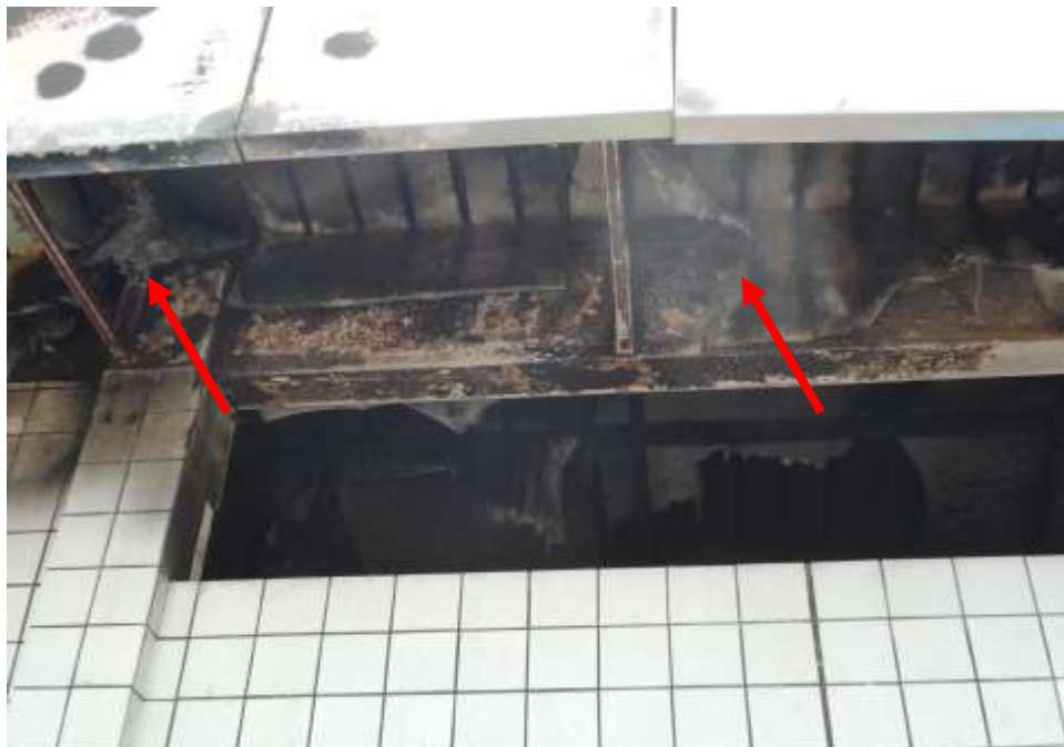
Photo 21 shows the fire damage on the roof linings. From our observations, the roof linings materials (arrowed) had caught fire and fall off the roof structure and onto the Insured Vehicle resulting the heat and smoke damage on the cabin top, resulting in high heat intensity burn marks (whitish burn marks) found on the exterior surface of its cabin top as well as rust.
