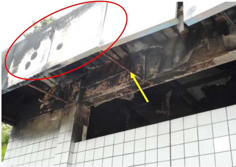
Photo 20 shows the fire damage on the roof panels. From our observations, the high heat intensity burn marks (whitish burn marks) found on the exterior surface of its roofs panels (circled) and rust that had developed on the metal support brackets of the roof panels (yellow arrow) on the structure of the rubbish collection centre.
