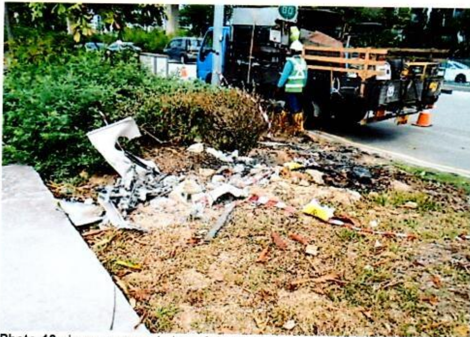
Photo 12 shows a general view of the burnt remains at the location where the electrical box was located. Repair/re-construction works to the electrical box and electrical cables were ongoing at the time of my inspection.
