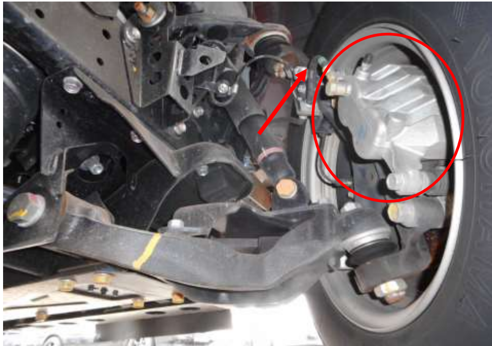
Photo 20 shows the brake hose/pipe (arrowed) at the front right wheel of the Motor Lorry. No leakage of brake fluid was observed. Visual examination of the various components of the braking system like the brake caliper (circled), brake booster, brake pedal etc had revealed all to be intact and without visible damage at the time of accident. There was also no sign of fluid stain(s) observed on the various undercarriage components.
