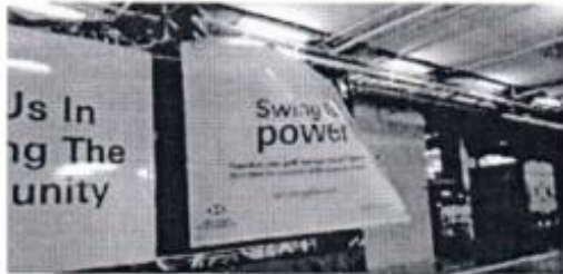
#Damages of the side panel – 3 out of 4 hinges was dislodged.
