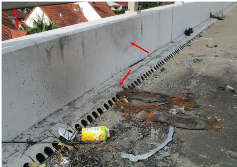
Photo 11 shows the burn marks on the adjacent kerb, barrier and railing nearest to where the Insured Vehicle was positioned when the fire occurred (arrowed).
