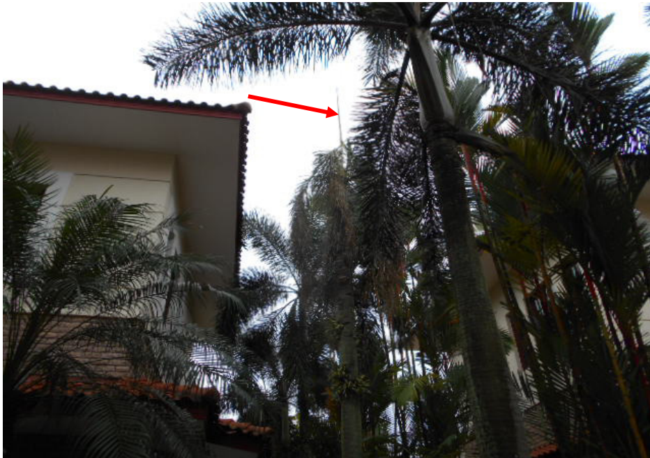
Photo 4 shows the sharp vertical pointed end (arrowed) of the tree that was stuck by lightning, as pointed out to me by Mr Tan. From a distance, this sharp vertical pointed end appears to be higher than the lightning conductors that were situation at the roof of the house.
