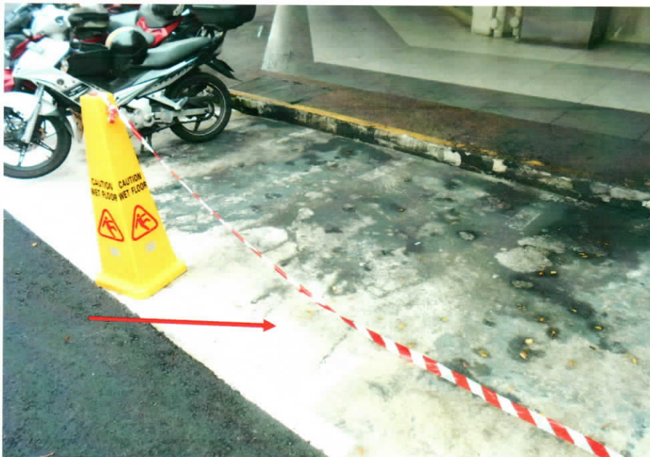
Photo 11 shows the burnt portion on the parking lot. We were able to clearly see burnt marks/ burned residual remains on the parking lot ground indicating that fire incident did took place at the said location.
