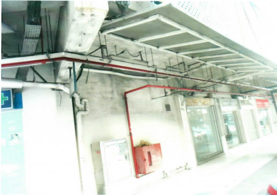
Photo 10 shows the burnt portion of the behind wall & ceiling indicates that fire incident did took place at the said location.
