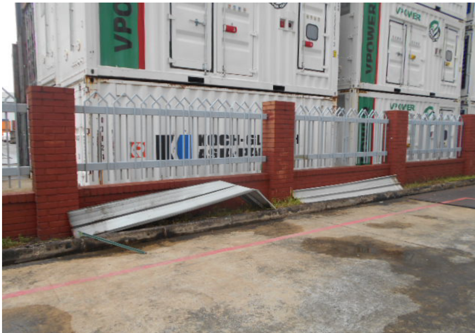
Photo 2 shows the 2 pieces of bent metal sheets that were initially lying on the driveway before being removed to the side to prevent obstruction to the driveway. These metal sheets were detached from the roof of a neighbouring warehouse by strong winds and blown to Toll Logistics premises at 17 Tuas Avenue 9.
