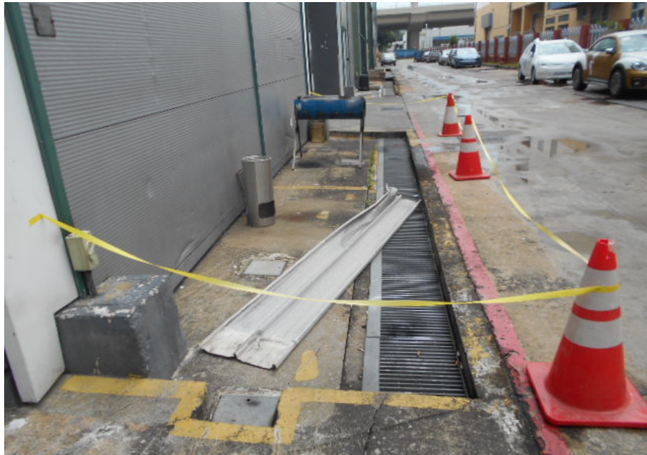
Photo 3 shows the bent metal sheet that was lying on the ground beside the building of Toll Logistics. This metal sheet was detached from the roof of a neighbouring warehouse by strong winds and blown to Toll Logistics premises at 17 Tuas Avenue 9. Glass shards were also found on the ground in the immediate vicinity of where this metal sheet was lying.
