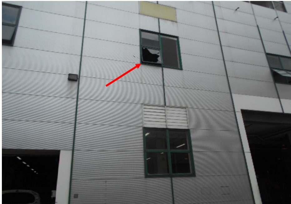
Photo 5 shows one of the building windows (arrowed) that was broken. This broken window was above the location where the single metal sheet and glass shards were found.
