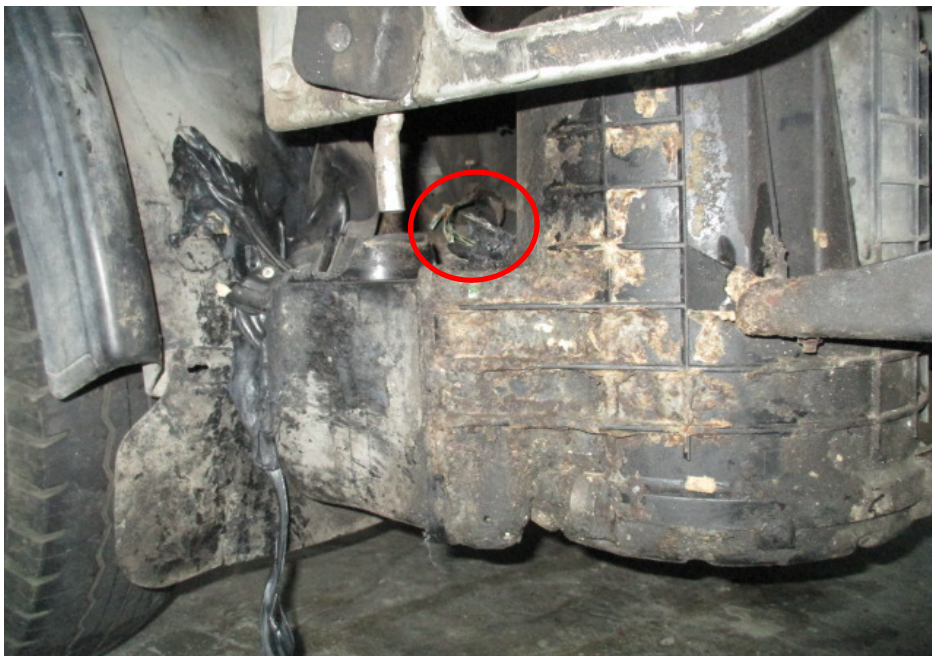
Photo 11 shows the burnt wirings of the Insured Vehicle's air cleaner assembly. We observed traces of greenish residue on some of these wirings (circled).
