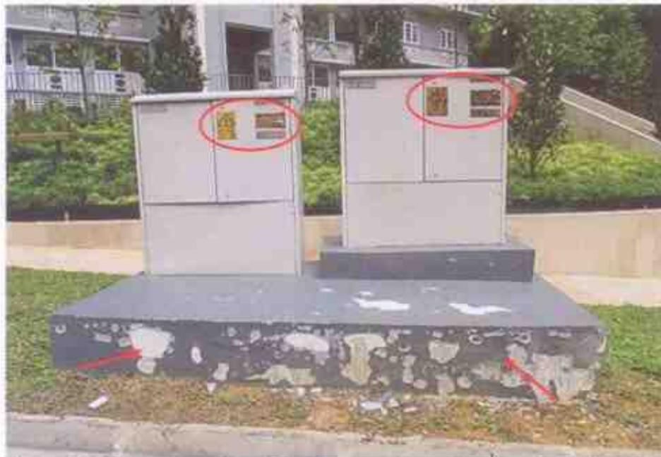
Photo 14 shows a closer view of the damage observed on the adjacent electrical fixtures. The paint is discoloured and flaky (red arrows). Bubbles have also formed on the warning and information signs due to exposure to prolonged high heat intensity from the fire (circled).
