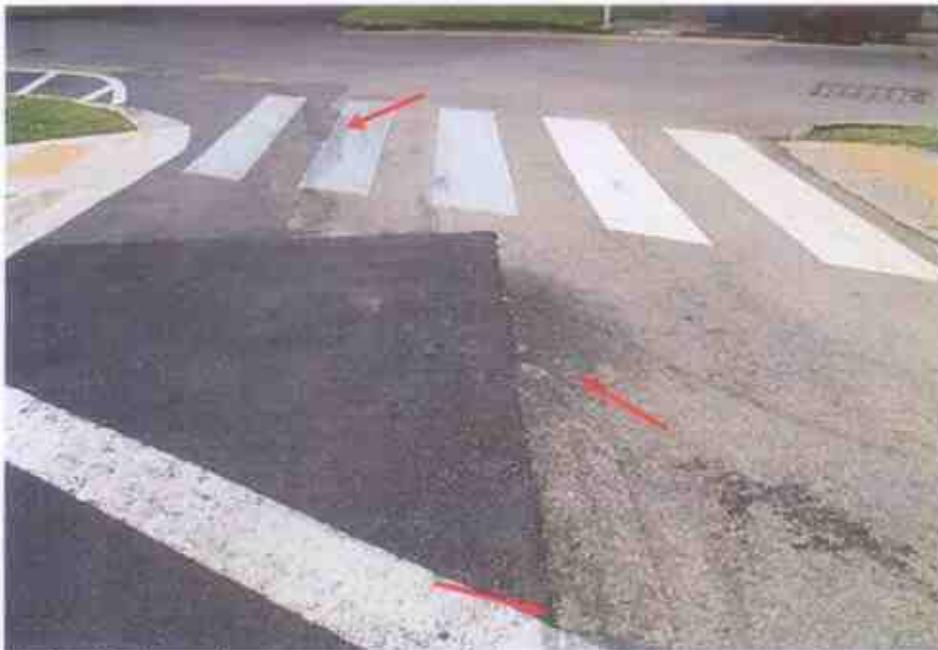
Photo 12 shows the burn marks and/or burnt residual remains on the ground before the filter lane into Sophia Road where the incident occurred (arrowed).
