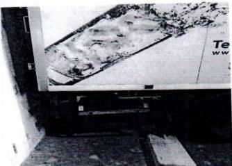
Photos of existing Vehicle stopper without color signage (for protection against property damages) and installed position is wrong, not able to protect the Electrical Riser Door!
