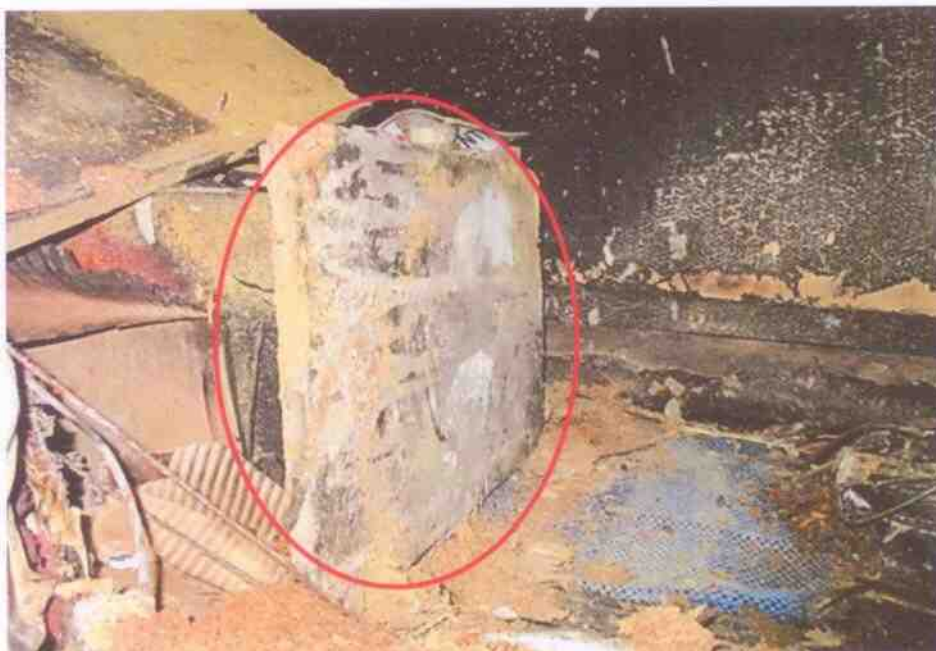
Photo 19 shows a closer view of the high heat intensity burn marks (whitish burn marks) found on the wooden shelves (circled) that were stored around the immediate vicinity to where the fire had likely started. These whitish burn marks are a result of exposure to prolonged heat intensity.
