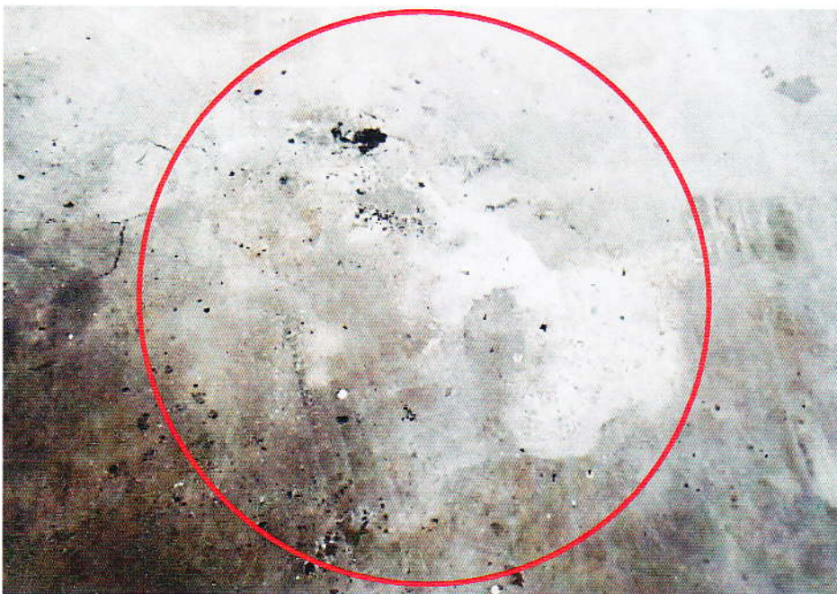
Photo 17 shows a closer view of the slight burnt marks and burnt residual remains (circled) that were found within the parking lot. This was towards the front centre of the parking lot, where the Insured Vehicle was parked.
