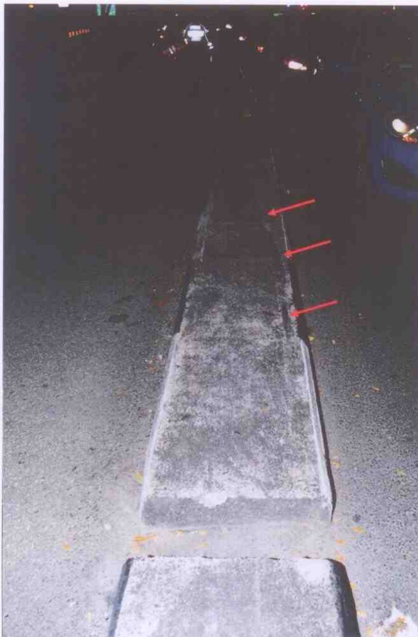
Photo 8 shows the stretch of centre divider road kerb from placard 5 leading to placard 6. Although not recorded by the police, I had observed what appears to be tyre marks (arrowed) on the top surface area leading towards placard 6.
