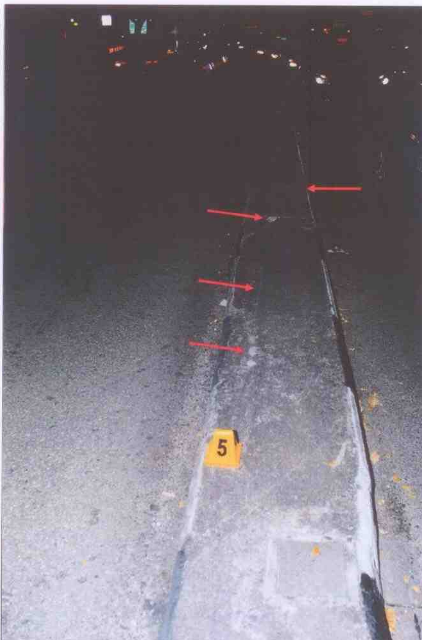
Photo 7 shows the start of placard 5, identified by the police to be gouge mark. Although the gouge mark was not clearly depicted in the photograph, I was still able to observe marks (arrowed) that appeared to be fresh, on the top surface of the centre divider road kerb.
