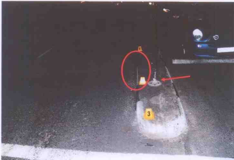
Photo 11 shows a general view of the centre divider kerb just after the pedestrian crossing. The Motor Car was likely to have mounted the centre divider kerb after placard 3, just before placard 5 (circled). The plastic bollard (arrowed), marked with placard 4, would have been possibly damaged by the Motor Car as it was mounting the centre divider kerb.
