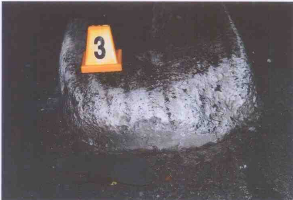
Photo 6 shows a closer view of placard 3, identified by the police to be chipped and scratch mark. I was not able to conclusively ascertain whether the chipped mark was a fresh damage or old damage. The lack of powdery residue surrounding the chipped off areas and/or on the road surface suggest that the damage to this part of the road kerb may have been not related to this accident.
