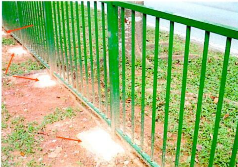
Photo 4 shows a close up view of the bases (red arrows) and the re-laid soil at the bottom of the greenish metal railings which are indications that these railings had been recently replaced.
