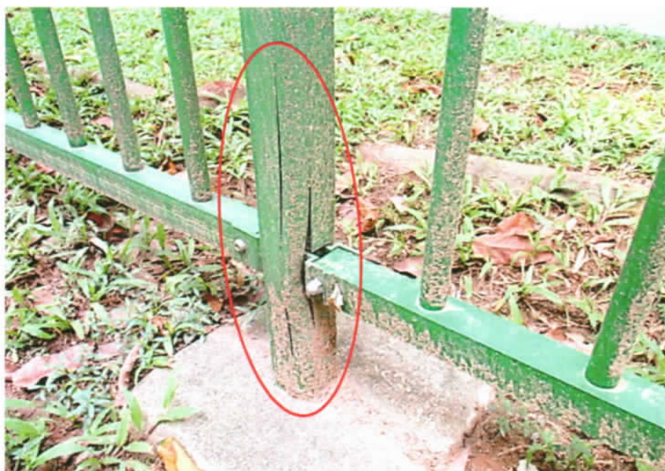
Photo 6 shows a close up view of the minor damage to the base of a railing (circled) adjacent to the tree Mr Chong had collided into.
