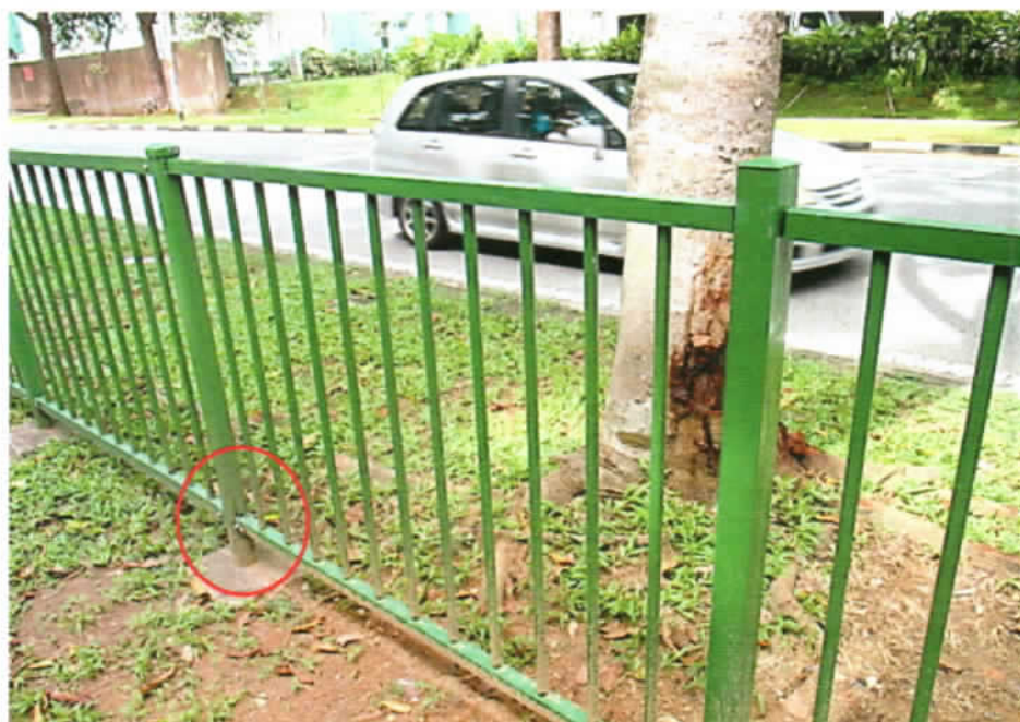
Photo 5 shows minor damage to the base of a railing (circled) adjacent to the tree Mr Chong had collided into.
