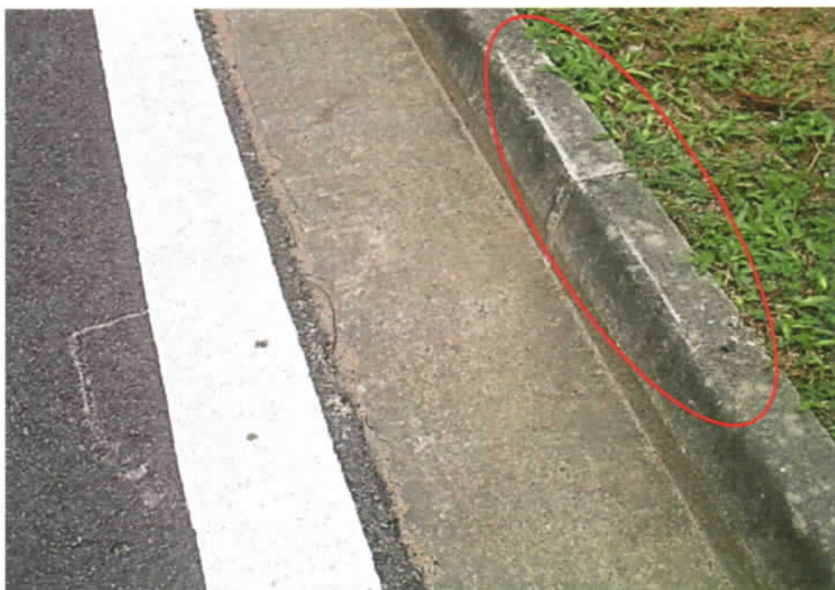
Photo 3 shows a close up view of the graze marks found on a kerb which Mr Chong had mounted (circled).
