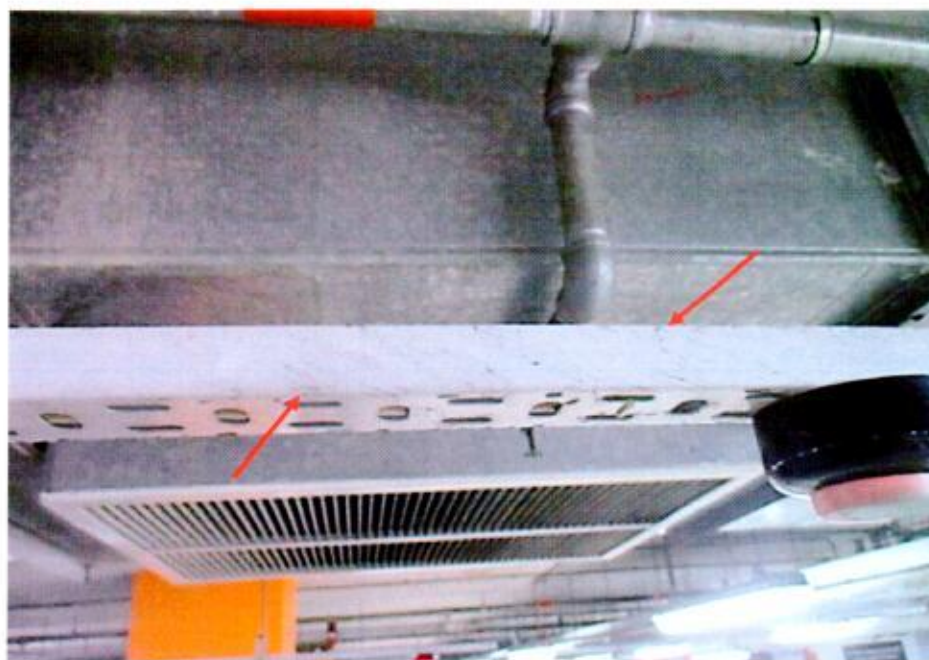
Photo 20 shows a close up view of a metal railing above the lot where the Insured Vehicle was parked blackened by soot (red arrows).
