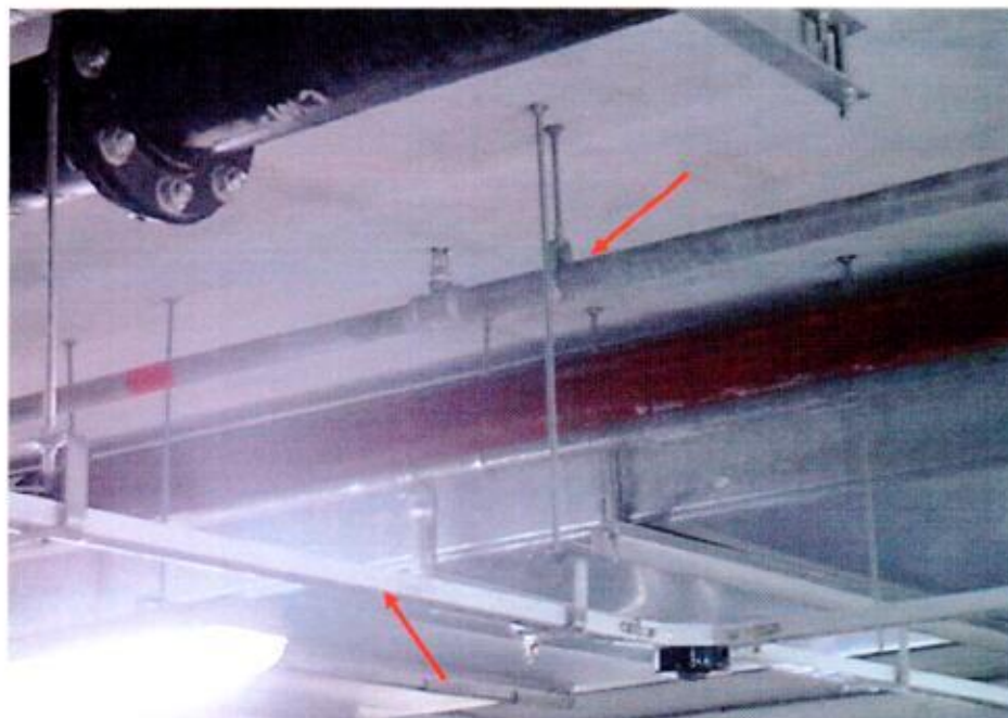
Photo 19 shows although we did not find any burnt marks and/or burnt residual remains on the ground where the Insured Vehicle was parked as there was a parked vehicle at the aforementioned lot at the time of our visit, we observed that the piping and metal railings above the lot where the Insured Vehicle was parked were blackened by soot (red arrows).
