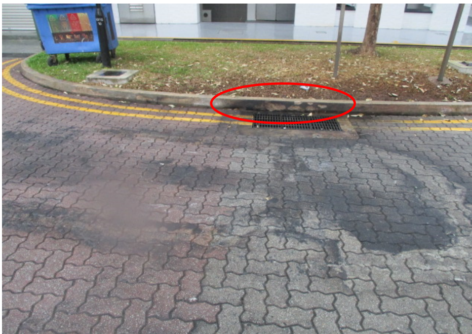
Photo 15 shows the burnt marks on the kerb nearest to where the Insured Vehicle was positioned when the fire occurred (circled). Apart from the burnt marks on the kerb, we did not observe any other damaged or newly replaced government property at the time of our visit to the incident location.
