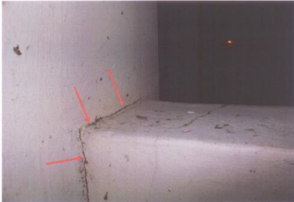
Photo 9 shows a single crack line (arrowed) formed between the perimeter wall and the pillar that was on the left side of the wall.
