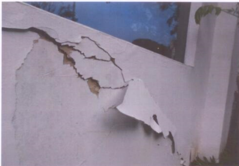
Photo 22 shows the single crack line on the interior side from the top surface stretching towards the bottom of the pillar at the right side of the wall.
