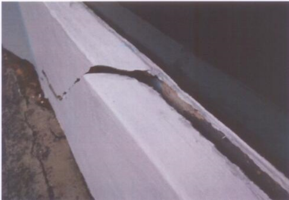
Photo 19 shows a section of the wall at the upper part and at the top surface, was separated into 2. The glass partition erected at the top surface of this wall was however unaffected.
