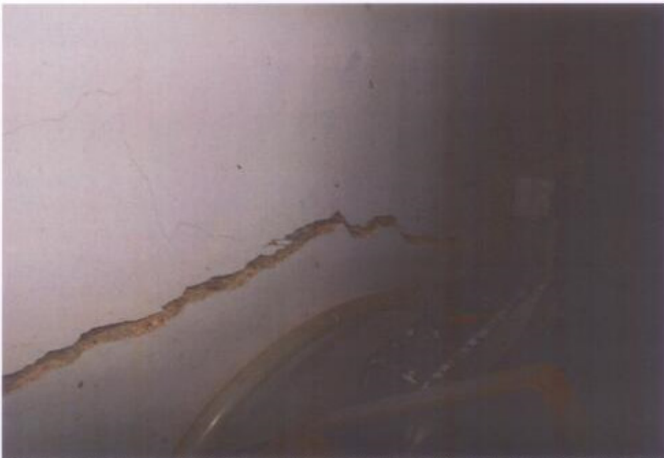
Photo 12 shows a closer view of the crack line on the interior side of the wall, leading towards the pillar on the right side of the wall.
