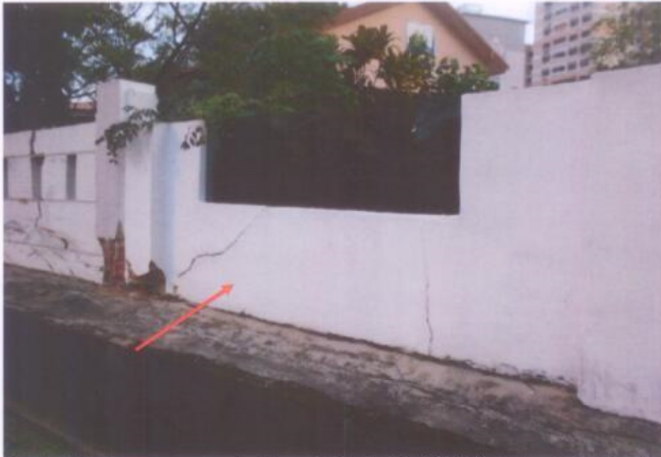
Photo 16 shows a general view of Block 46 #01-190 Jalan Bahagia. The perimeter wall (arrowed) towards the right of the unit (from the perspective when standing inside the unit) was observed to have been damaged on its exterior side and interior side. The pillar at the right side of the wall was also affected. The glass partition erected at the centre section of this wall was however unaffected.
