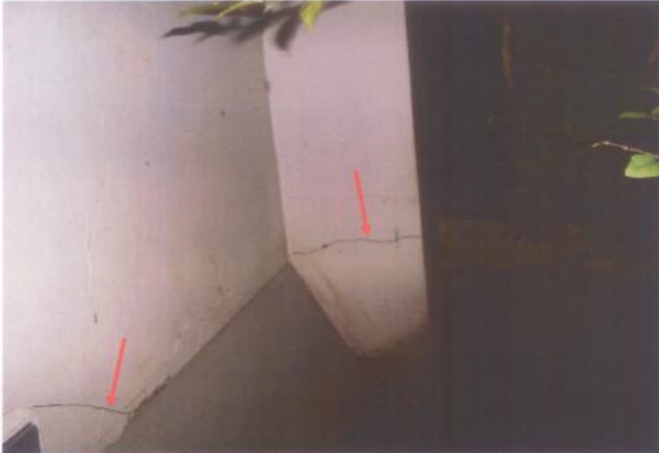
Photo 13 shows a single crack line (arrowed) on the interior side of the wall, leading towards the pillar on the right side of the wall.
