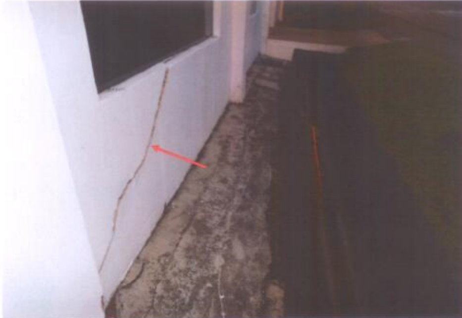
Photo 18 shows the single crack line (arrowed) on the exterior side of the wall, from the pillar extending towards the upper section of the wall.
