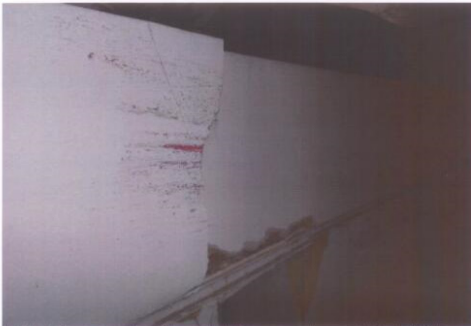
Photo 6 shows a section of the wall at the upper part separated into 2. This was on the exterior side of the wall.
