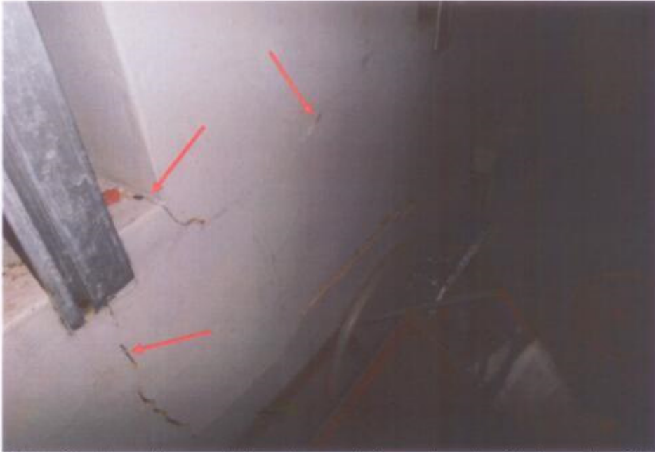
Photo 11 shows the crack lines (arrowed) formed on the interior side of the perimeter wall. The crack lines were largely traced from the exterior side of the wall extending into the interior side.
