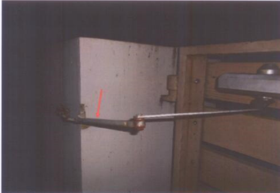
Photo 15 shows the horizontal holding arm (arrowed) of the gate, which was mounted on the pillar towards the right of the wall. Due to slight shifting of this arm, the horizontal bolt of the access gate could not slide into its lock chamber.
