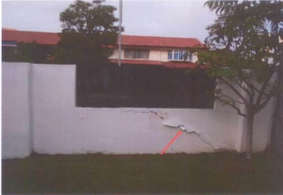
Photo 20 shows a general view of the interior side of the damaged perimeter wall of Block 46 #01-190 Jalan Bahagia. A single crack line (arrowed) was observed on the interior side from the top surface stretching towards the bottom of the pillar at the right side of the wall.
