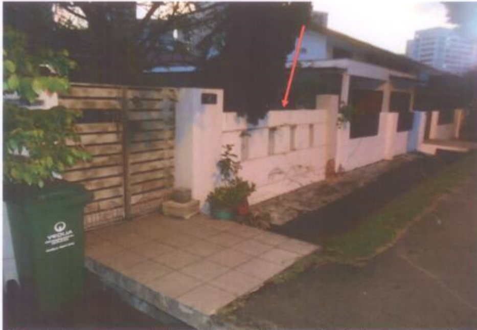
Photo 1 shows a general view of Block 45 #01-192 Jalan Bahagia. The perimeter wall (arrowed) towards the left of the unit (from the perspective when standing inside the unit) was observed to have been damaged. The 2 pillars at the right side and left side of the wall, together with the access gate of the unit were also affected.
