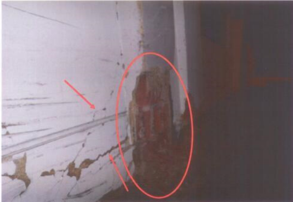
Photo 5 shows the crack lines (arrowed) of the wall extending towards the pillar at the left side of the wall. The cement at the base (circled), on the exterior side of the pillar, was also observed to be broken, exposing the bricks used to construct the pillar.
