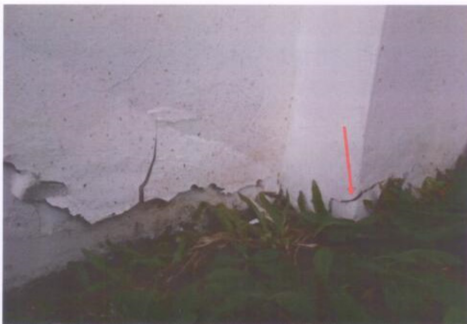
Photo 23 shows the single crack line on the interior side from the top surface stretching towards the bottom of the pillar (arrowed) at the right side of the wall.
