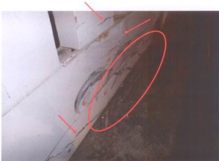
Photo 4 shows a closer view of the damage to the exterior side of the perimeter wall. Multiple crack marks (arrowed) were seen on the wall. The base of the wall (circled) was also observed to have been shifted inwards.
