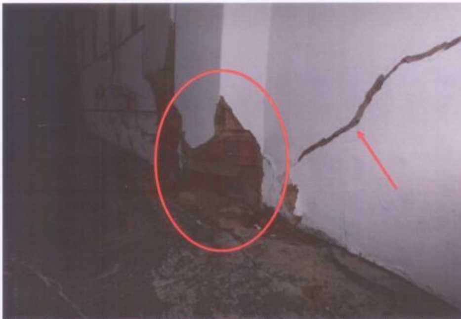
Photo 17 shows the cement at the base (circled) on the exterior side of the pillar broken, exposing the bricks used to construct the pillar. A single crack line (arrowed) was formed from the pillar extending towards the upper section of the wall.
