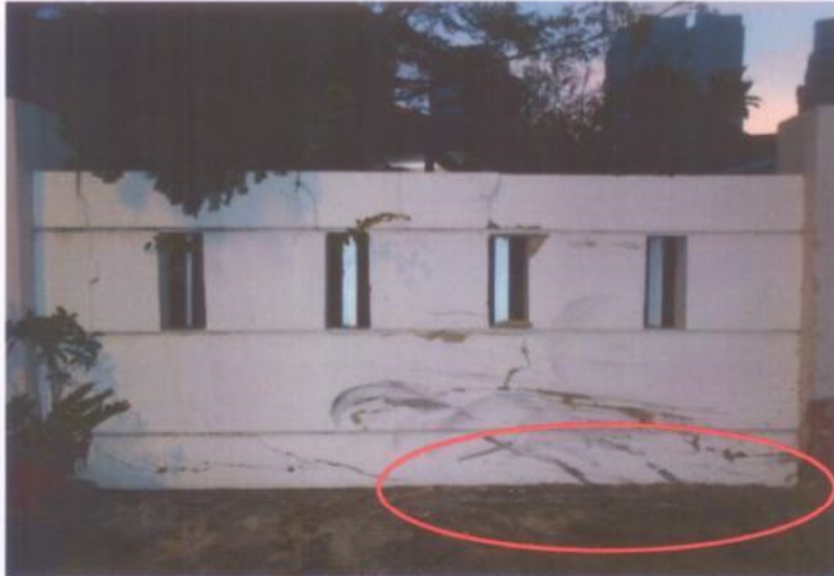
Photo 3 shows a general view of the damaged perimeter wall of Block 45 #01-192 Jalan Bahagia. The wall was found to be with multiple crack lines. The crack lines could be found on both the interior side and exterior side of the wall. The base of the wall (circled) was also observed to be shifted inwards.
