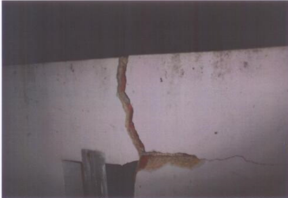
Photo 7 shows a section of the wall at the upper part separated into 2. This was on the interior side of the wall.
