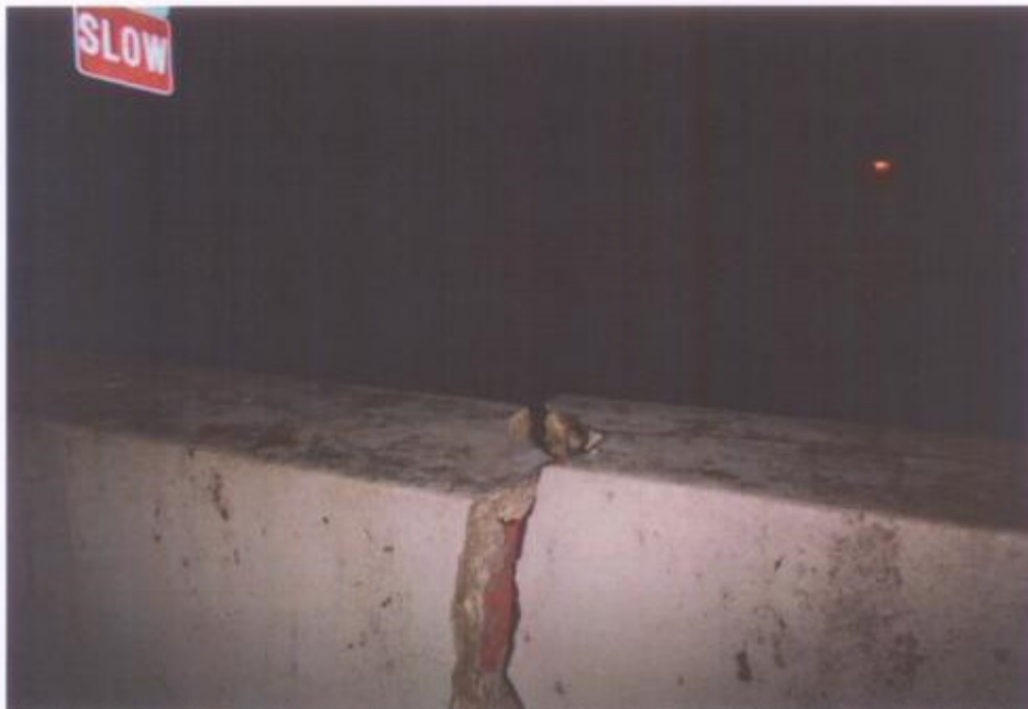
Photo 8 shows a section of the wall at the upper part separated into 2. This was at the top surface of the wall.
